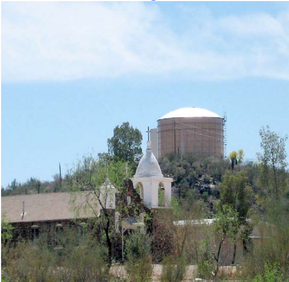
Photograph-Sells Water Storage Tank
